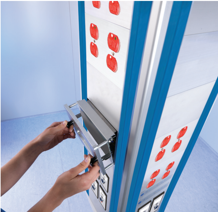
Removal of supply module with a Trumpf Medical extraction tool.
